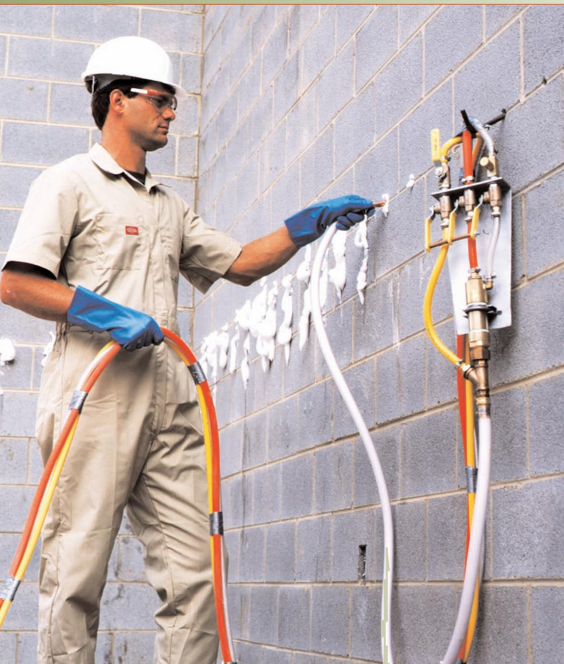
Core-Fill 500™ is a thermal and acoustical amino-plast masonry foam insulation with superior R-values, excellent sound absorption characteristics and enhanced fire-safety performance.
