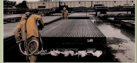
Hollow-core, pre-stressed concrete panels.
